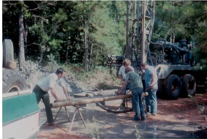
Figure 12 – Coring Operations to Evaluate Uranium Mineralization and to Characterize Aquifers Above and Below Mineralized Zones
