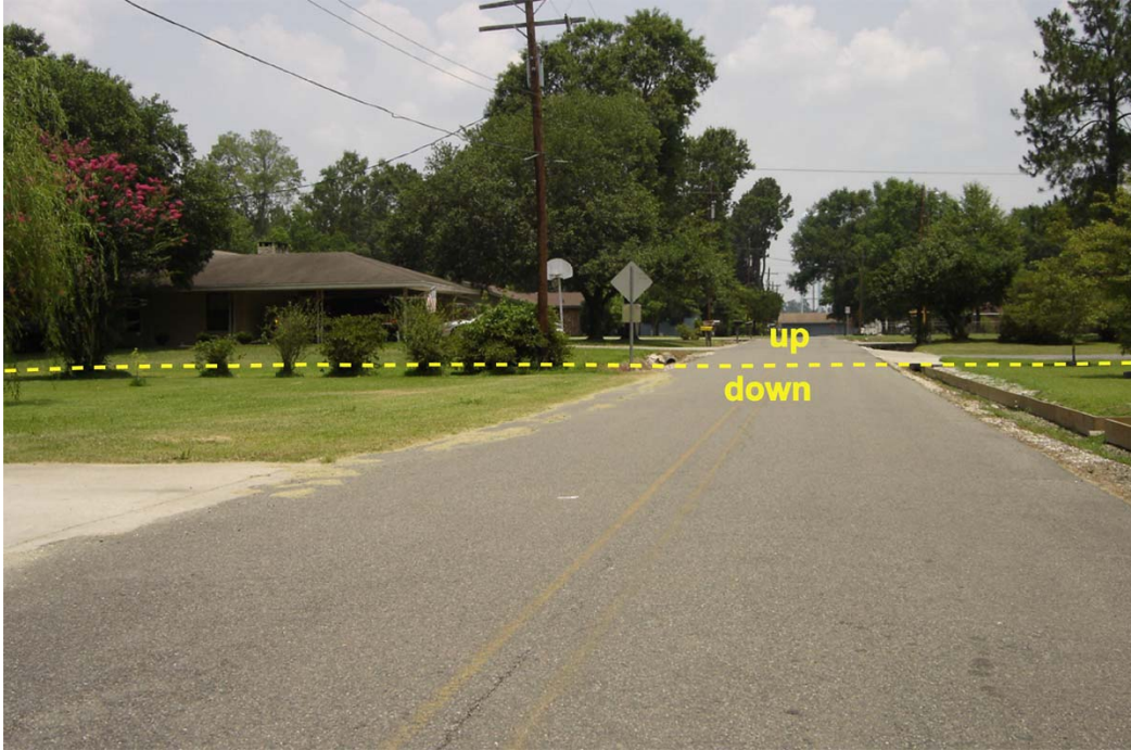
Figure C.5. Photo of the Moss Bluff fault-related step near Moss Bluff. The dashed line represents the approximate location of the fault trace.
