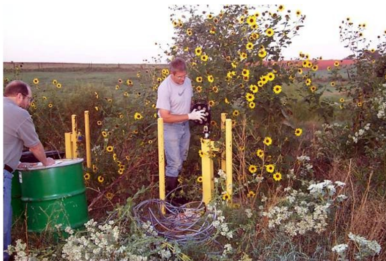
Typical Monitoring Wells (Deep and Shallow)
