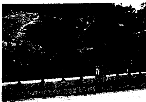
Figure 2.2.2.6 Road cutting in thrust fault in gneiss-granite, Stockholm. The fault zone is about 0.2 m thick and consists of gravelly, crushed rock. High storativity. Note the seepage of water on the left side of the picture (black colour of the rock).
