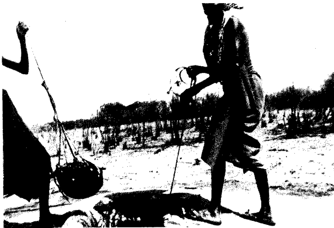
Figure 3.3.1.1 Women drawing water from a traditional hand-dug well lined with bent branches to retard or prevent caving. The hole is circular, and about one metre in diameter. Note that the well mouth is reduced in size by rectangularly-placed logs, notched by many passages of bucket ropes. Some wells of similar construction are about 0.80 metre across. Buckets are constructed of circular-cut skins attached to strings, a design permitting them to lie flat on the bottom of the well.
